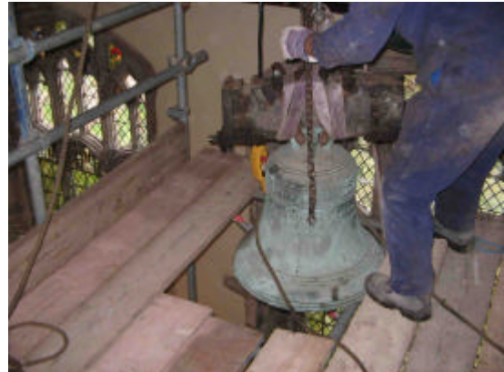
Nettlestead's new treble awaits hanging (above left) whilst the refurbished number 2 bell is hauled up the scaffolding before being swung across and lowered into its pit (right).
